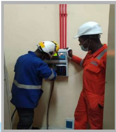
Complete Procurement, Installation & Commissioning of VESDA VLC ASD at Yokri -SPDC
