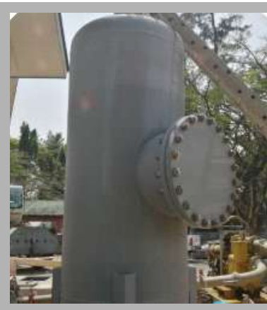
Installation and commissioning of knockout drum and activated vessels
