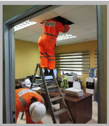
Installation of multiple units of addressable fire alarm system integrated to a central com system- Geometric power plant
