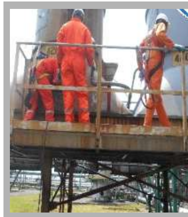
Hydro jet cleaning of a gas heat exchanger unit at OB-OB Facility
