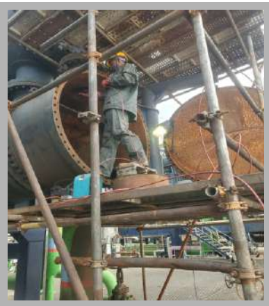
Online Cleaning 120 Units Of Shell & Tube Heat Exchangers at Dangote Refinery 200,000 Tubes Approx
