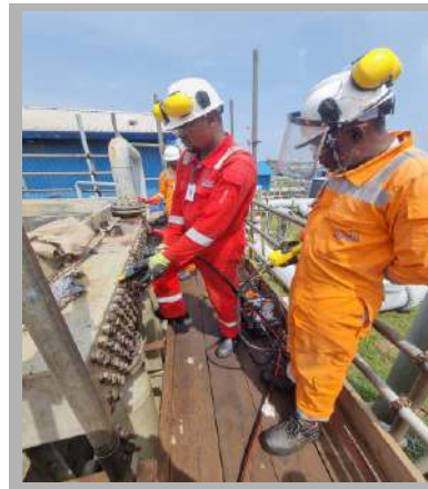
Onsite Hydraulic Bolt Torquing Activity at QIT -SEPNU
