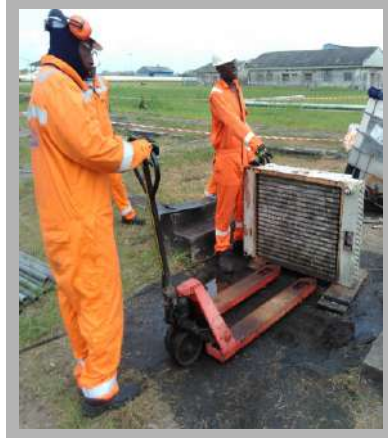
HEX Leak Test & Tubes Cleaning On Leaking Condensate MLP-102a Cooler
