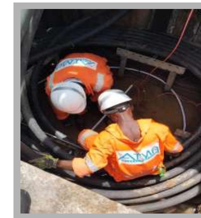
33KVA Cable Trunking at Aba power
