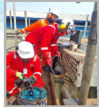
After clean inspection with our VBS-30 Video scope and probe
