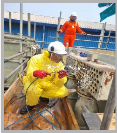
Intrusive Cleaning And Tube Plugging Of Cooper #2 Heat Exchanger At Qua Iboe Terminal
